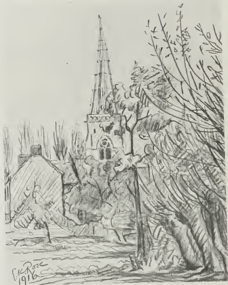
RCBECQ FROM THE SOUTH.
